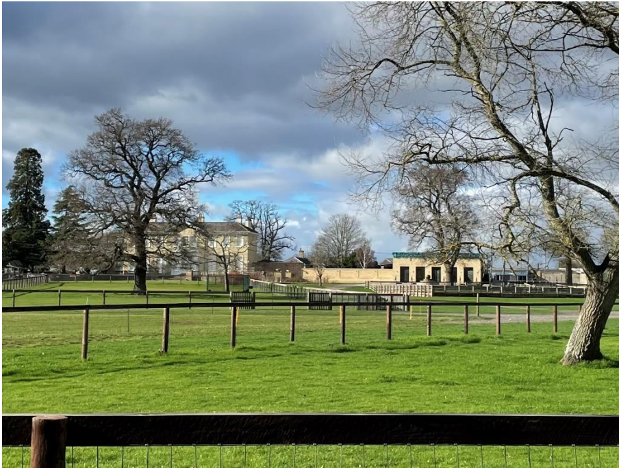
Plate 16: 2024 image of the as-built pool house and wall.
